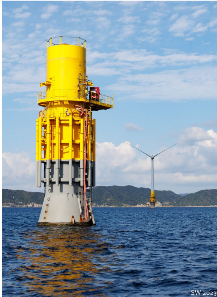
Offshore wind farm under construction using spar buoy type foundations, Goto Islands, Nagasaki Prefecture
