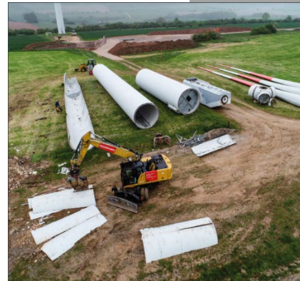
Decommissioning of Onshore Wind Turbines
